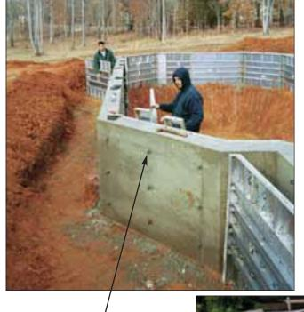
The exposed tie ends are easily broken off using a standard hammer or the Swim-crete Tie Breaker Bar.
