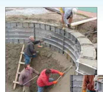
Concrete is placed into the concrete forms at a 3" slump starting in the deep end walls. Once deep end walls are filled with concrete, the walls are vibrated; this allows concrete to flow under interior forms. Next placement continues in the deep end of the pool, stacking concrete until both wall and floor come together achieving monolithic pour.
