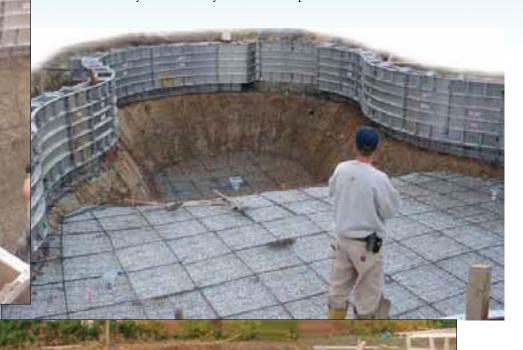
3" (8 cm) slump recommended for all-concrete monolithic pool pours.
